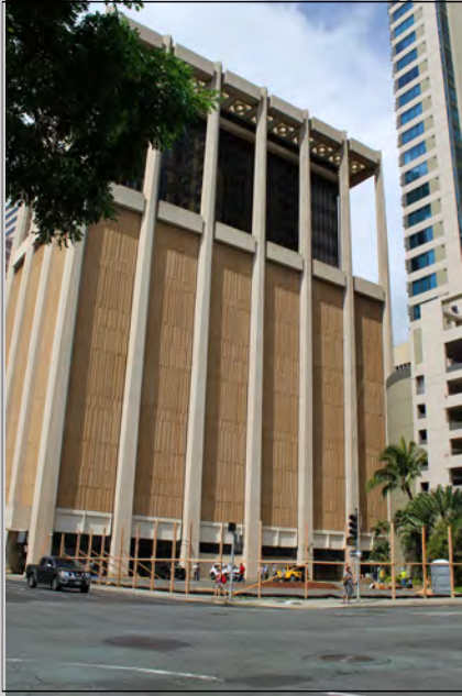
Kokua groundbreaking, September 2021
