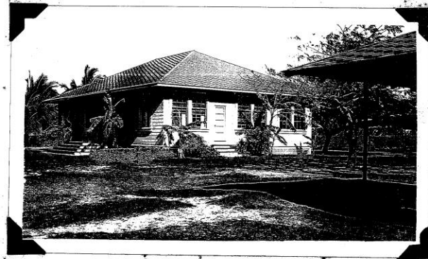
SUPERVISING PRINCIPALS' OFFICE
