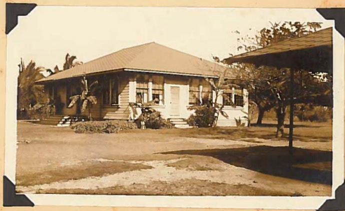
SUPERVISING PRINCIPALS' OFFICE
