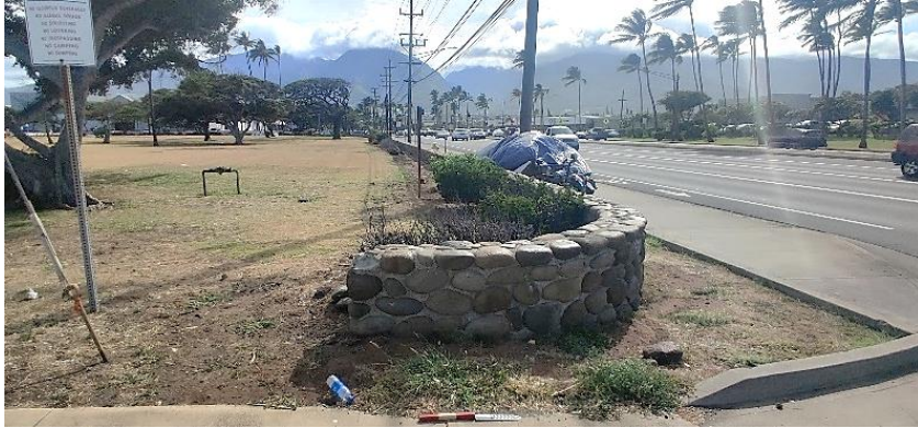
Figure 26. Eastern extension, facing west.
