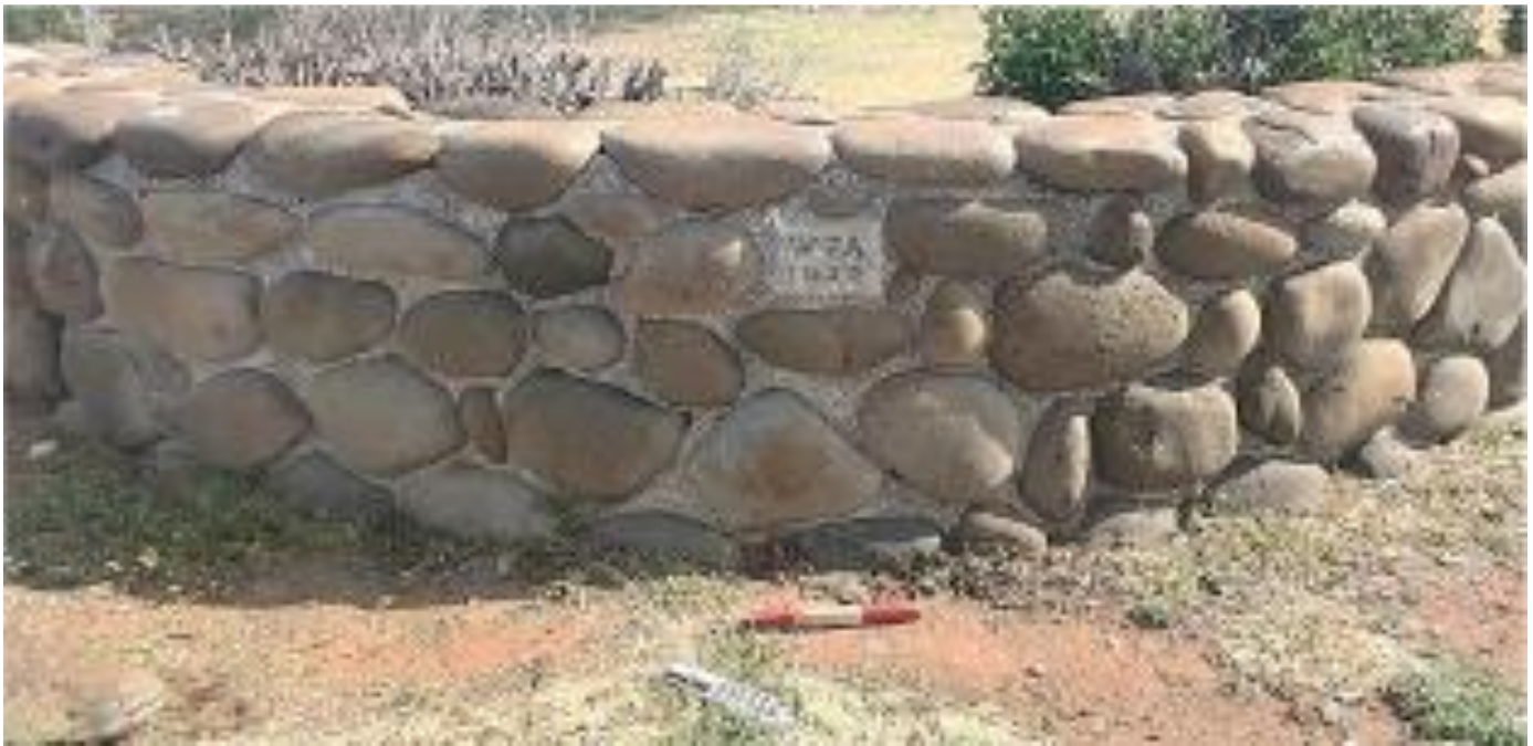
Figure 9 Stone and mortar wall with embossed date of construction, "WPA 1939." (Photograph courtesy of Keala Pono Archaeological Consulting 2021)
