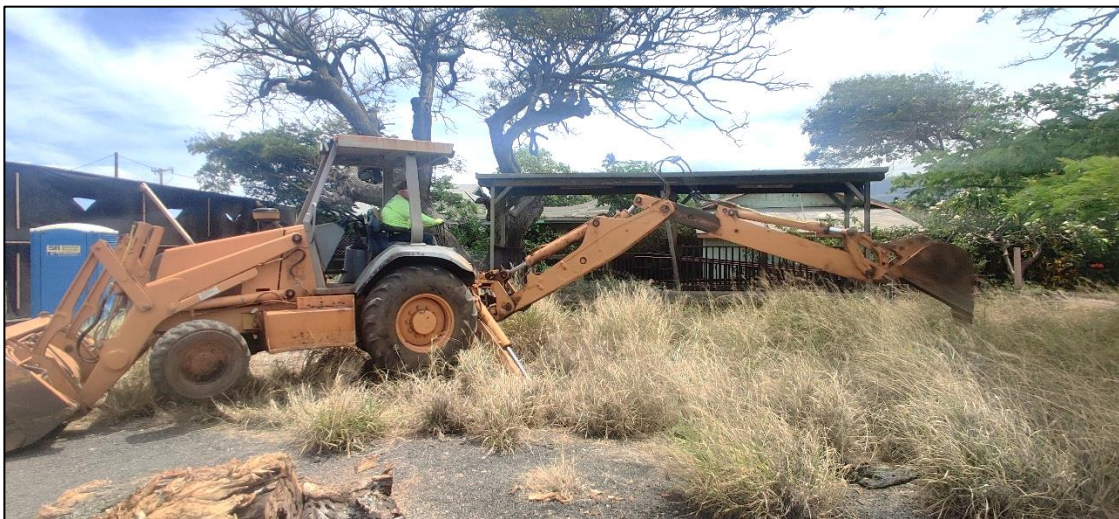
Figure 16. Excavation with a backhoe. Orientation is to the southeast.
