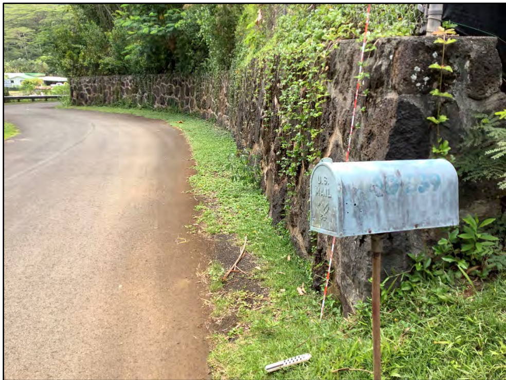
Figure 79. CSH 14, mortared basalt retaining wall with metal fence, view to west (CSH 2022)
