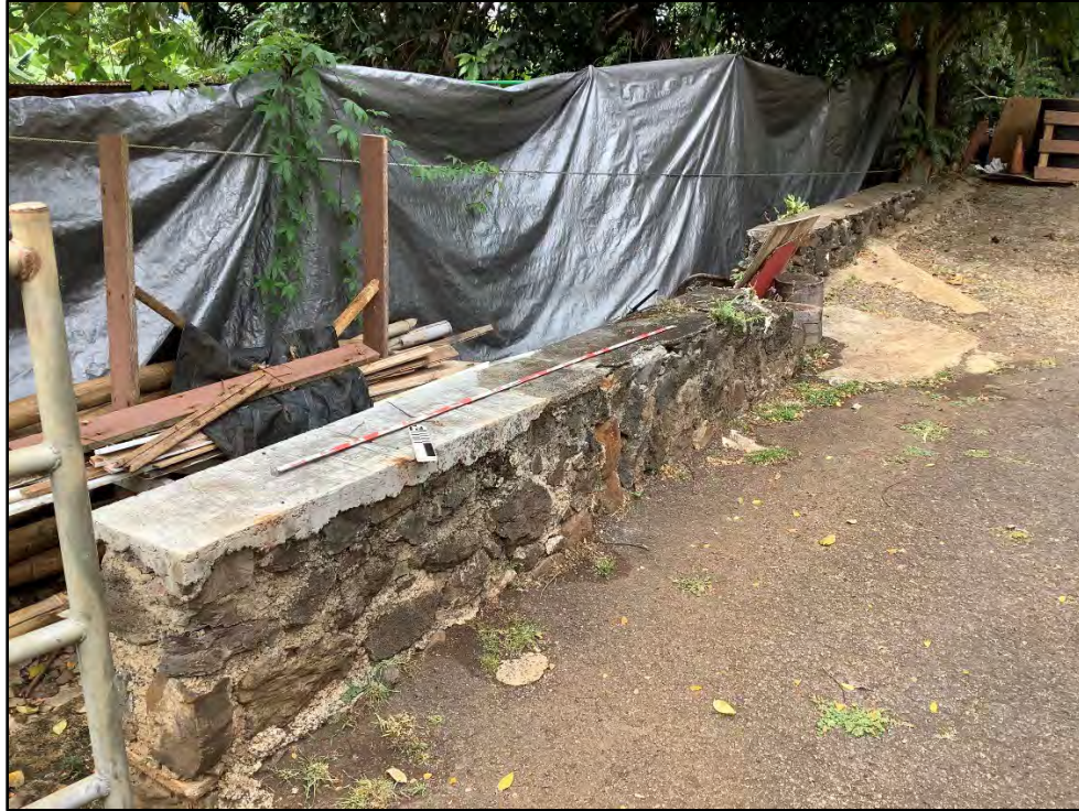
Figure 97. CSH 30, mortared basalt retaining wall, view to north (CSH 2022)
