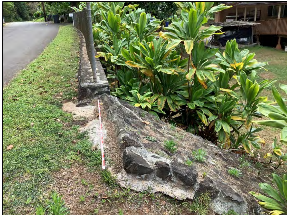
Figure 96. CSH 29, mortared basalt retaining wall with downslope portion, view to west (CSH 2022)
