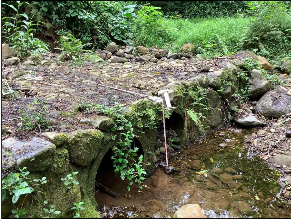
Figure 76. CSH 12, mortared basalt bridge/culvert spanning Uwau Stream, view to north (CSH 2022)
