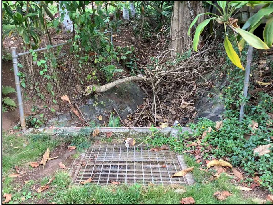
Figure 95. CSH 28, mortared basalt culvert, view to southwest (CSH 2022)
