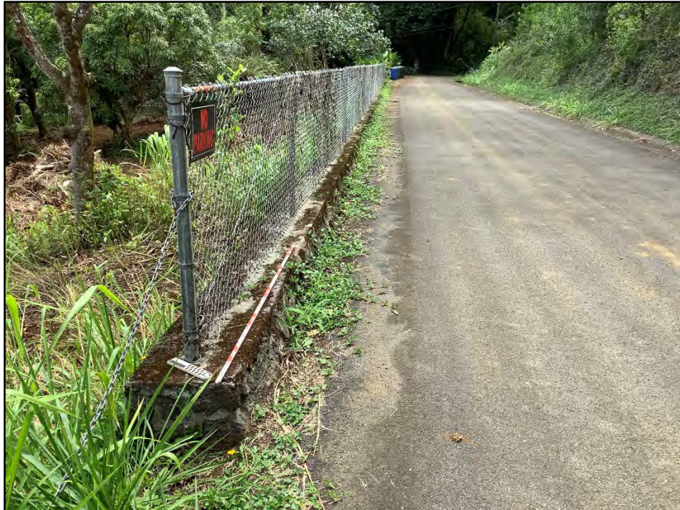
Figure 82. CSH 16, mortared basalt retaining wall, view to southwest (CSH 2022)
