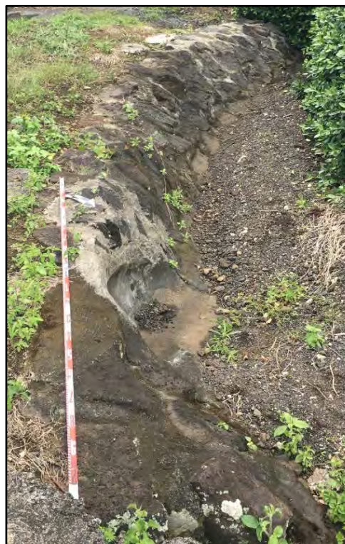
Figure 65. CSH 5, mortared basalt culvert on the northwest corner of the Waiāhole Valley Road–Kamehameha Highway intersection, view to southwest (CSH 2018)
