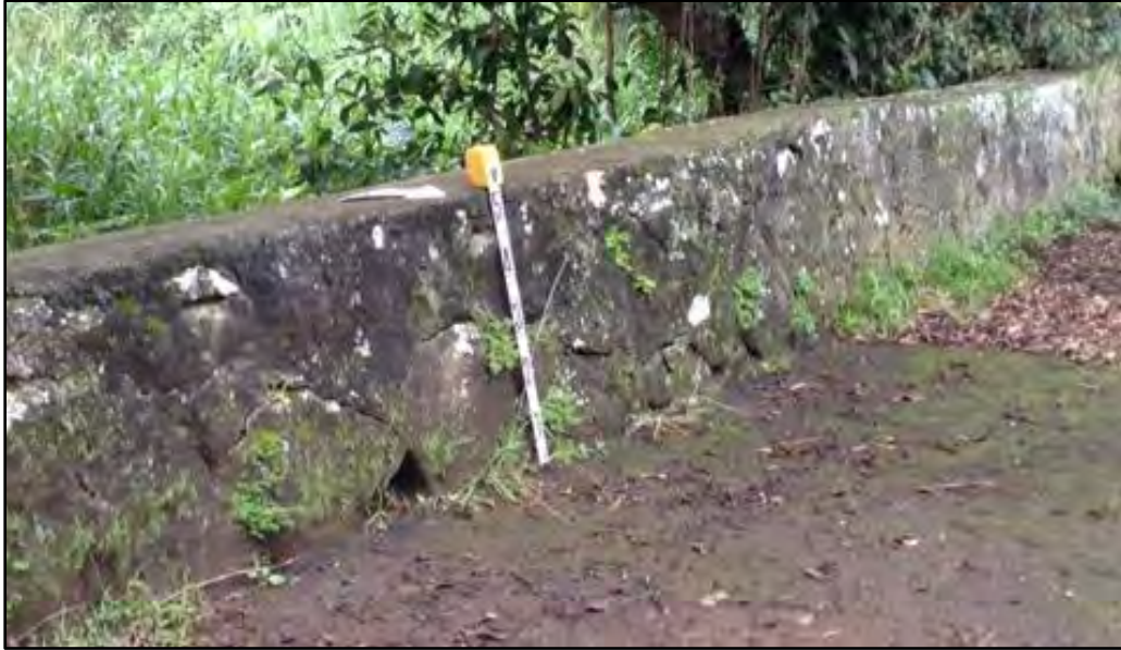
Figure 58. CSH 1 Feature C, mortared basalt retaining wall on the south side of Waiāhole Valley Road, view to southwest (CSH 2018)
