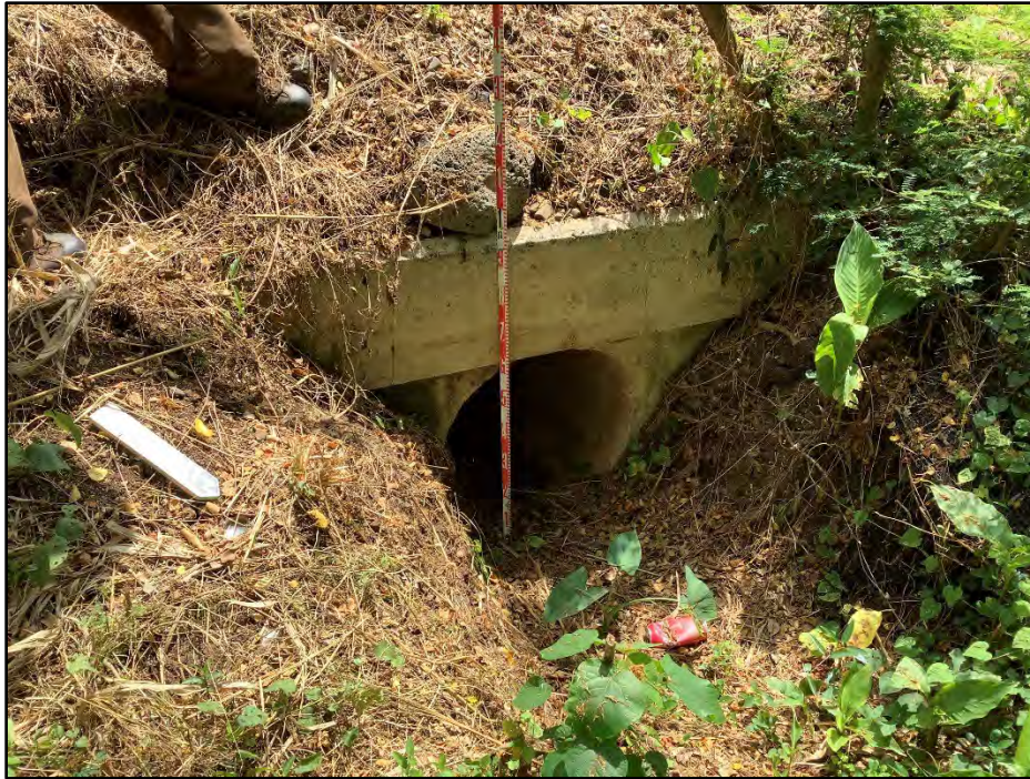
Figure 99. CSH 31, concrete culvert outlet on opposite side of Kamehameha Highway from mortared basalt portion, view to southeast (CSH 2022)
