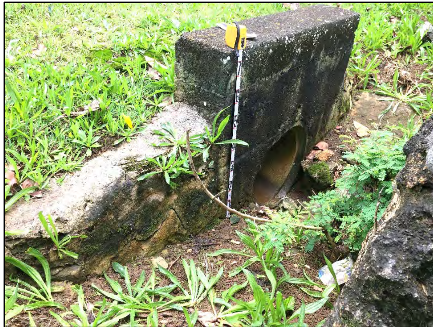
Figure 62. CSH 2 Feature A (concrete culvert, center) and Feature B (mortared basalt retaining wall, right) from the opposite angle, view to southwest (CSH 2018)
