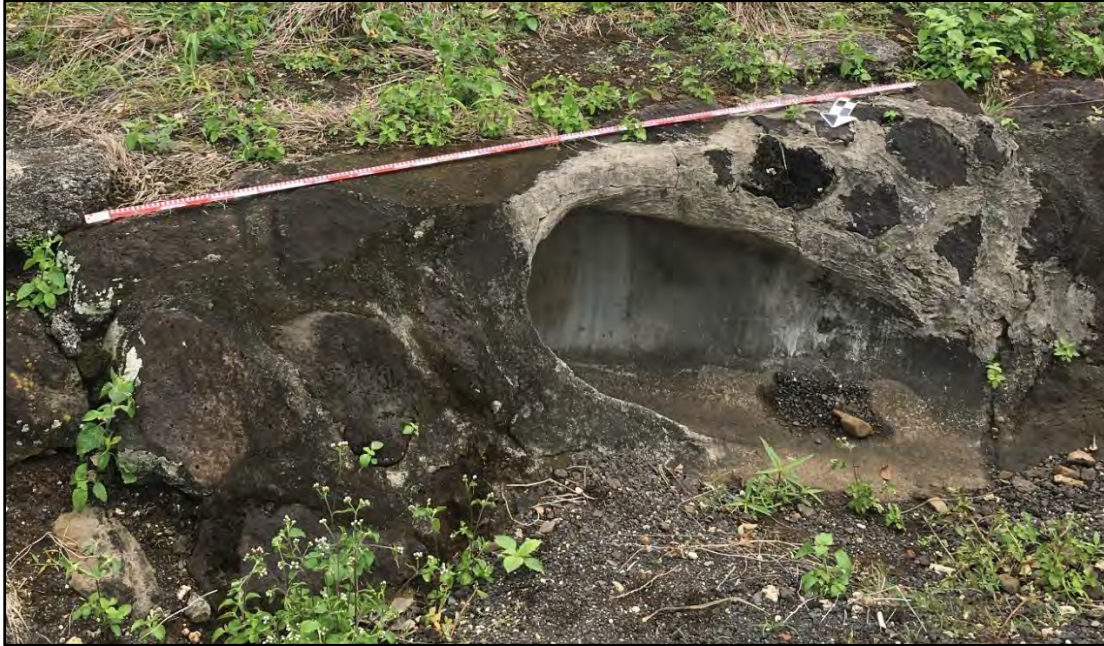
Figure 66. Close-up of the east end of CSH 5, mortared basalt culvert, showing the ca. 50-cm diameter opening, view to southeast (CSH 2018)
