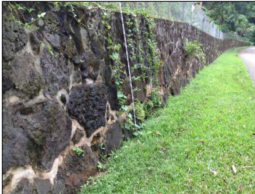
Figure 64. CSH 4, mortared basalt retaining wall on the south side of Waiāhole Homestead Road, view to southwest (CSH 2018)
