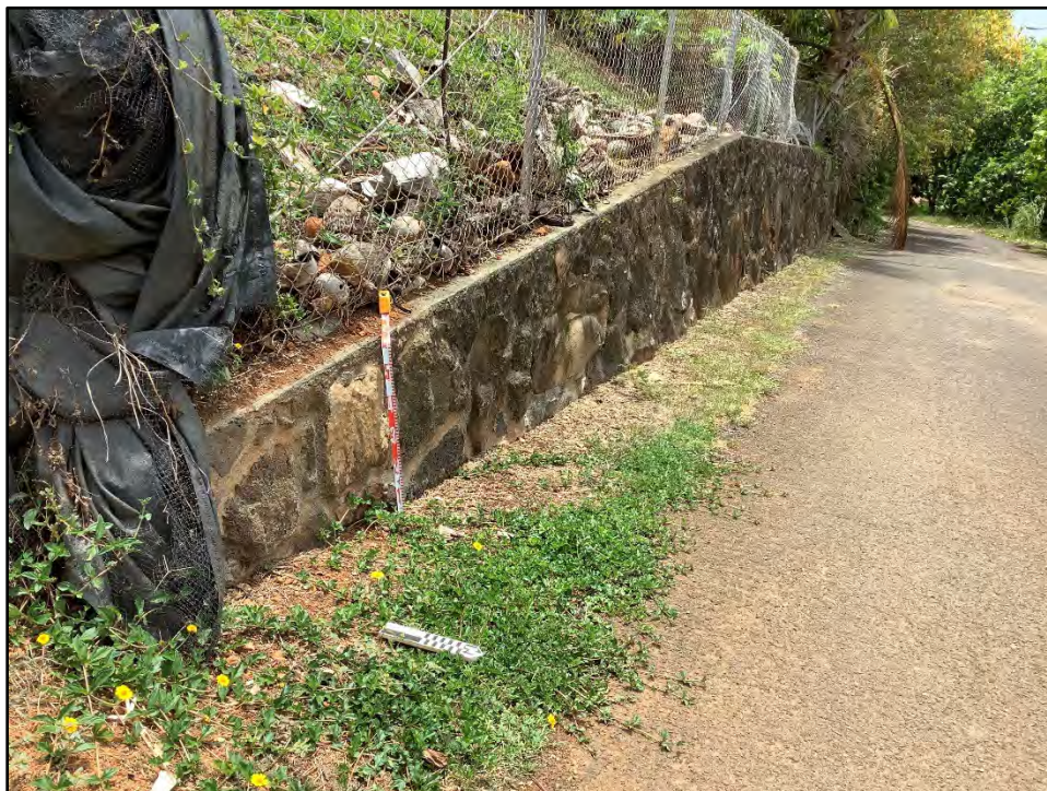
Figure 92. CSH 25, mortared basalt retaining wall, view to west (CSH 2022)
