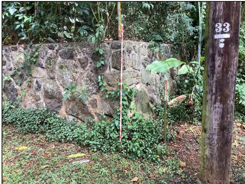
Figure 87. CSH 22, mortared basalt retaining wall, view to west (CSH 2022)
