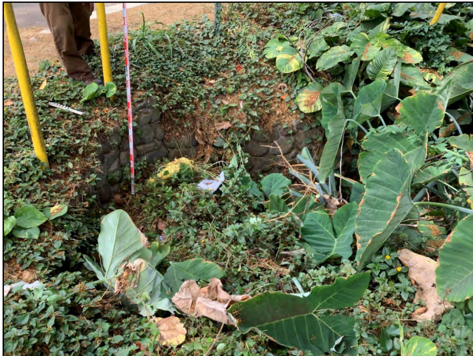
Figure 98. CSH 31, mortared basalt culvert, view to east (CSH 2022)
