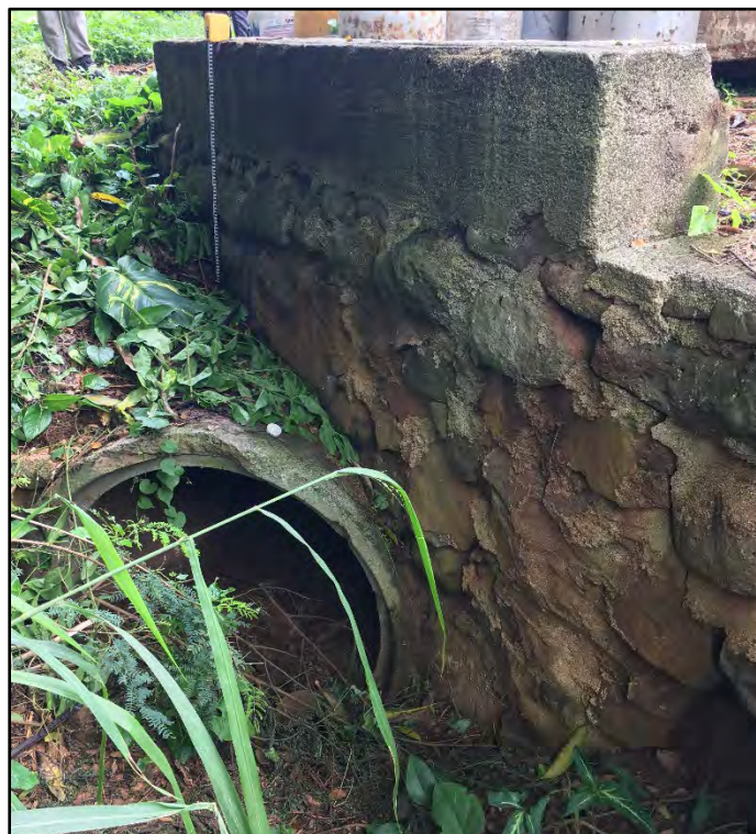
Figure 63. CSH 3, concrete and mortared basalt culvert on the north side of Waiāhole Homestead Road, view to southeast (CSH 2018)
