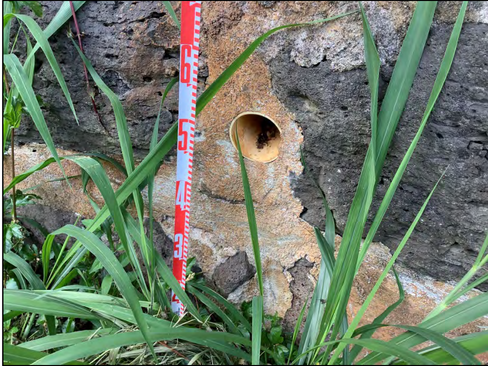
Figure 80. CSH 14, close-up of PVC drainage pipe near base, view to northwest (CSH 2022)
