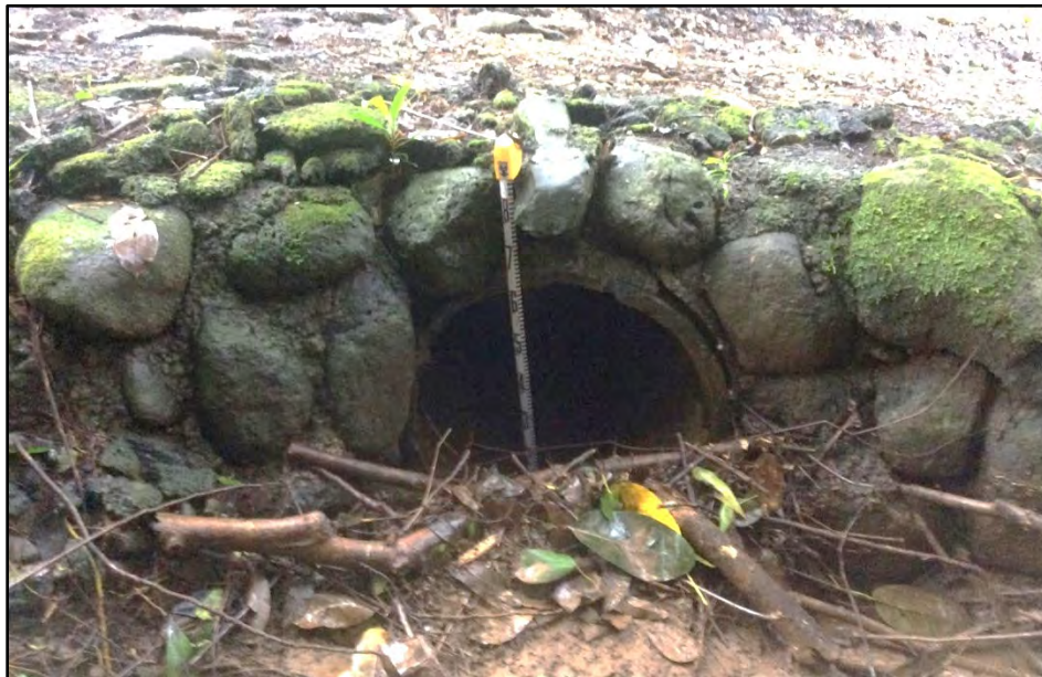
Figure 69. North portion of CSH 8 Feature A, mortared basalt culvert with concrete pipe, view to south (CSH 2018)
