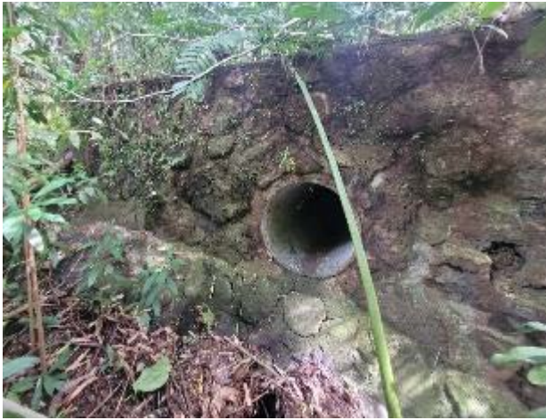
The road's storm water system discharge.
