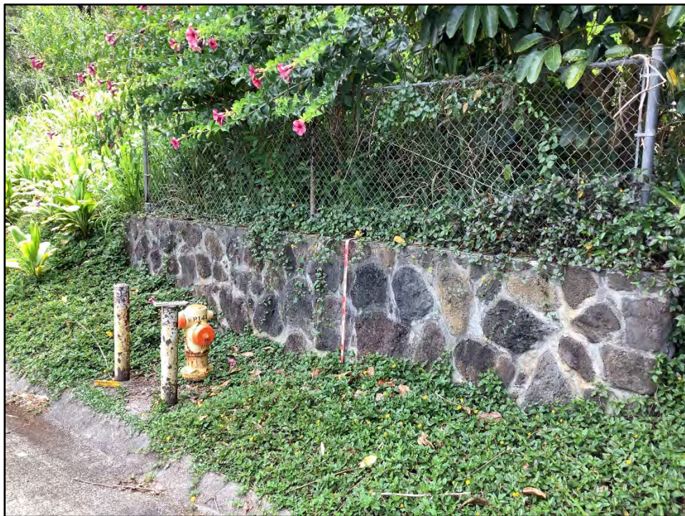
Figure 81. CSH 15, mortared basalt retaining wall, view to west (CSH 2022)
