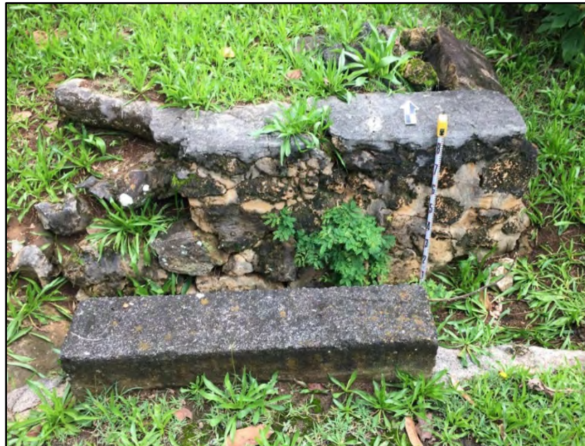
Figure 61. CSH 2 Feature A (concrete culvert, bottom) and Feature B (mortared basalt retaining wall, top) on the north side of Waiāhole Valley Road, view to north (CSH 2018)
