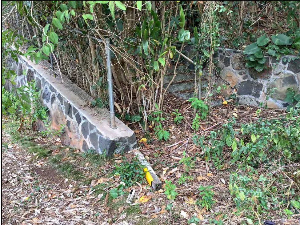
Figure 93. CSH 26, mortared basalt retaining wall with staircase, view to south (CSH 2022)
