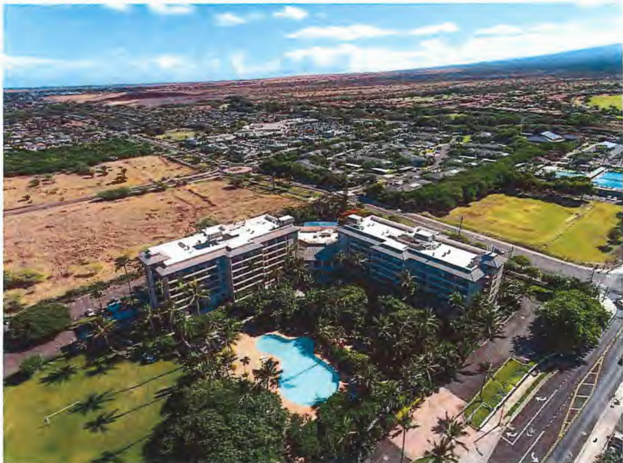
Northeast Aerial View
